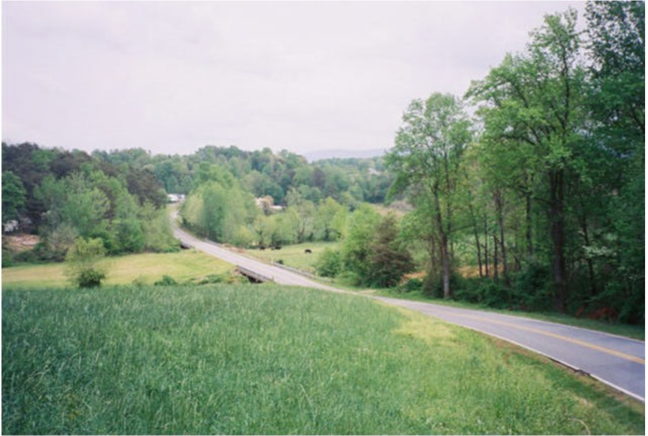
Patton Rd. Facing Southeast to Silver Creek (first bridge) and Hall Creek (second bridge)
